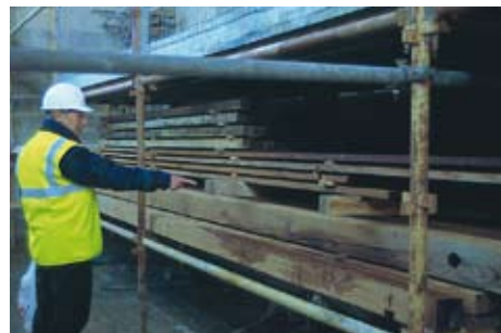
Reclaimed timber stored on site
