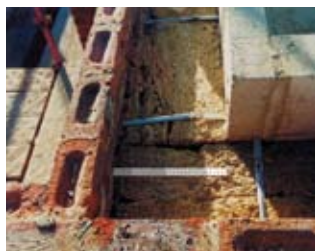
Super-insulation with wall tie
